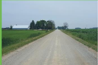
90 MW Proposed Windfarm Bad Axe, MI (Deerfield II)
